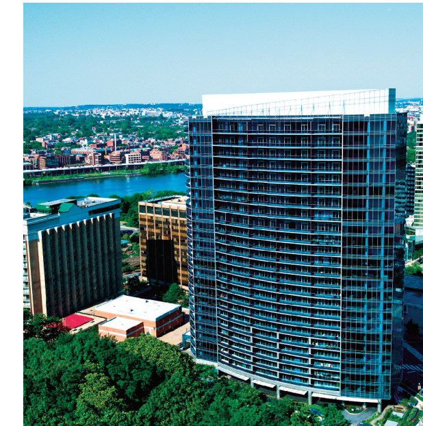
TURNBERRY TOWER ARLINGTON, VIRGINIA
