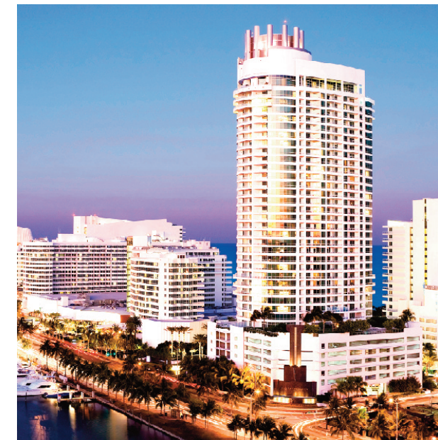
FONTAINEBLEAU TRESOR TOWER, MIAMI BEACH, FLORIDA
